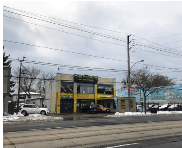
Subject site, looking southwest
