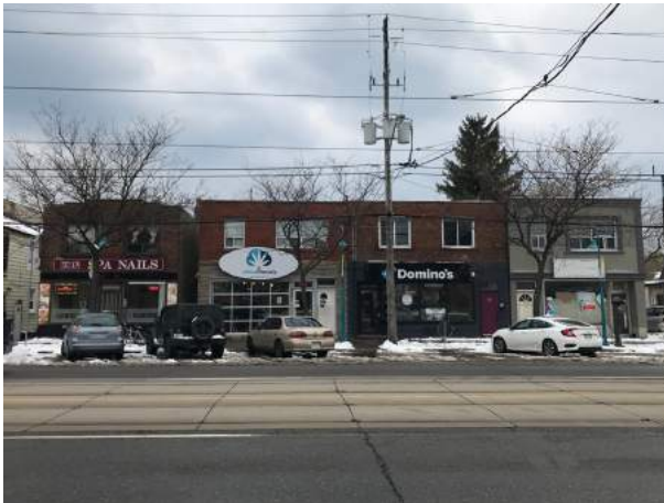
3351 – 3339 Lake Shore Boulevard West
