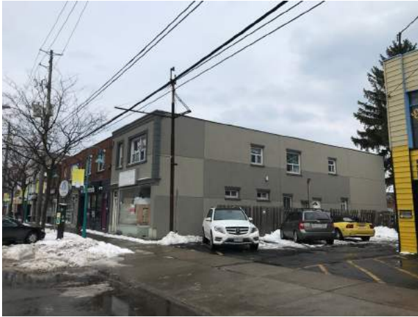
3351 Lake Shore Boulevard West (westerly building façade) looking southeast
