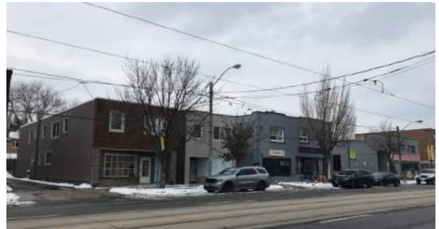
Commercial mixed-use buildings along Lake Shore Boulevard West (3366 – 3392 Lake Shore Boulevard West, looking northeast)
