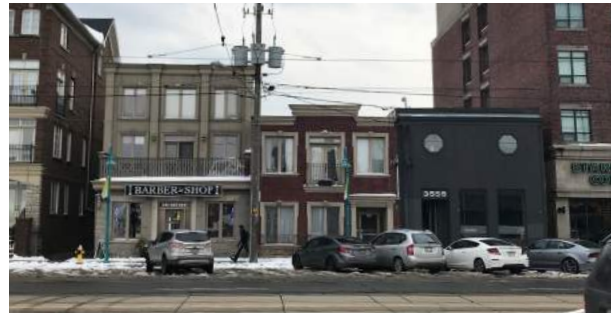
3545 – 3555 Lake Shore Boulevard West
