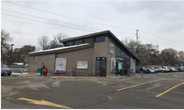
Long Branch GO Station (Long Branch Loop)
